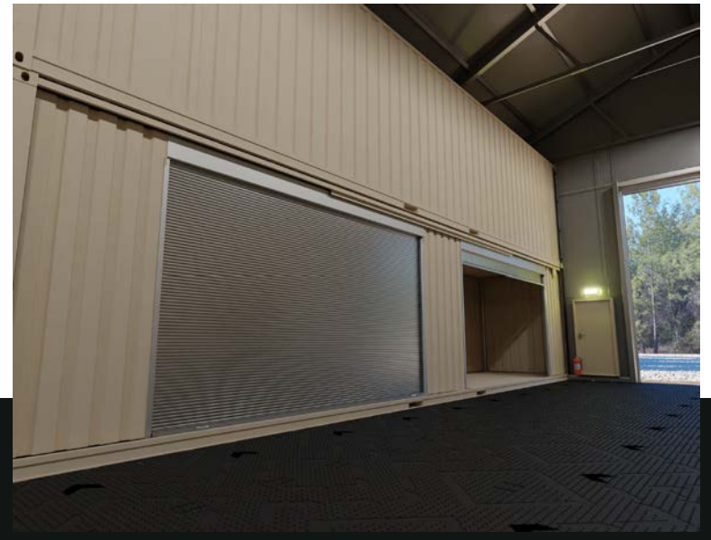
RACKBOX SHELTER interior. 40 ft modified container with roller shutter access
